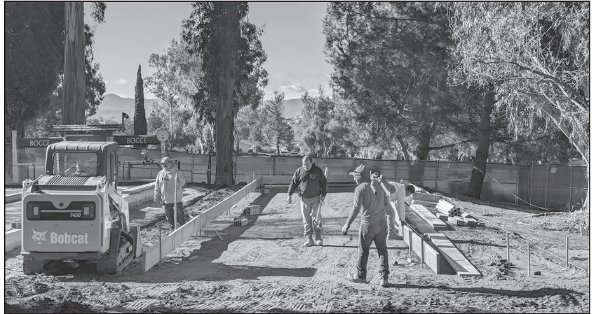
Good weather equals good progress for bocce court #3.
