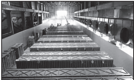
Battery racks sit in former turbine halls at Moss Landing Energy Storage Facility
