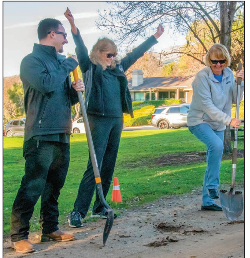
The ceremonial groundbreaking for The Villages' third Bocce court took place Friday, January 5. Kicking off the construction project are (Shown left to right) Ryan Bell, Jana King and Judy Owen. (See more photos of the event on page 9).
