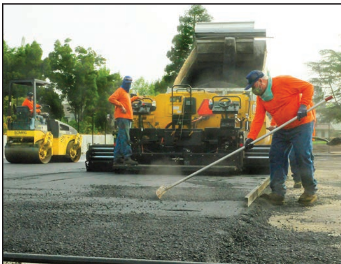
September 15—Courts paved with asphalt
