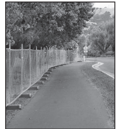
The temporary construction fence went up August 5.
