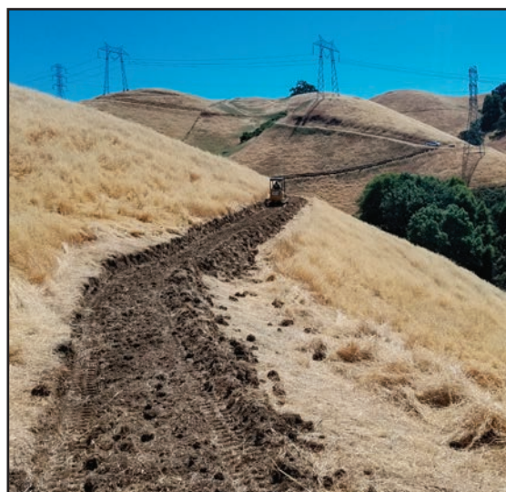
Workers regrading and widening a trail.
