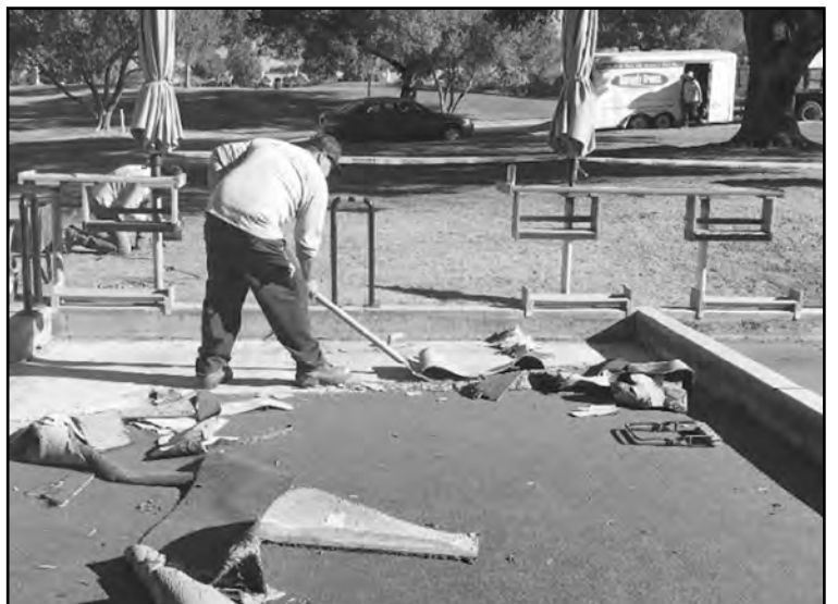
Starting carpet removal November 5 on Court #2 by Heavenly Greens.
