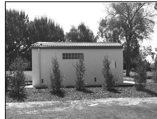
New restroom on Hole 17.
